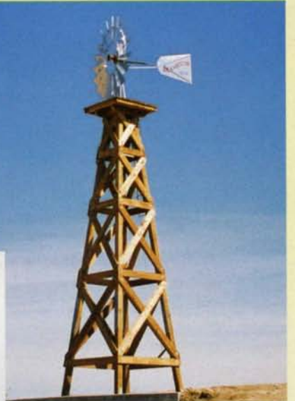
8' Mill on a 33' Platform/ Western Red Cedar Tower - Strasburg, Colorado
