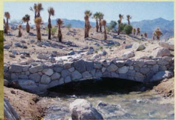
Arch Plate Series 20' Clear Span x 12' Wide 10,000# Vehicle Loading
