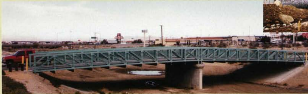
Entrance to Tanger Factory Outlet Mall, Barstow, CA 2 x 14' W x 135' L with 4' W Pedestrian Access Way.
