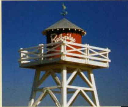
25' H Water Tower Platform, Redbridge Development
