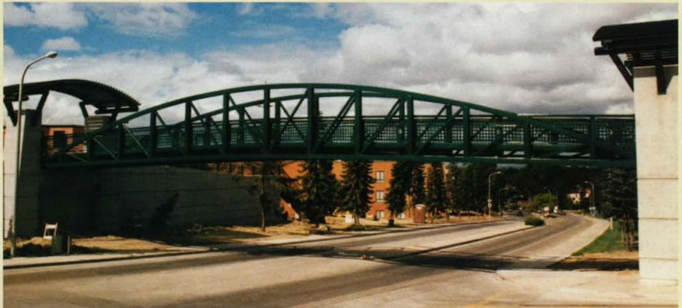
Bow Truss configuration, University of California, Irvine 14' W x 103' L 20,000 lbs. vehicle capacity
